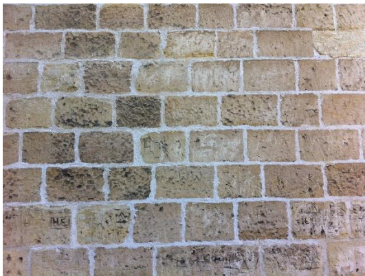
Lime mortar pointing
