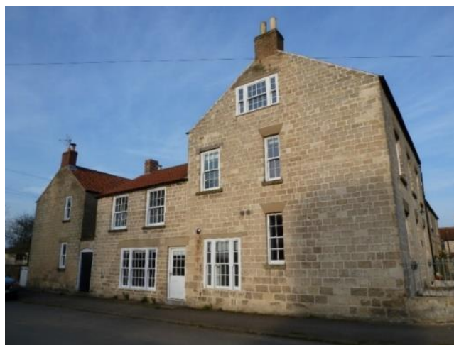
Lime pointing at Prospect House
